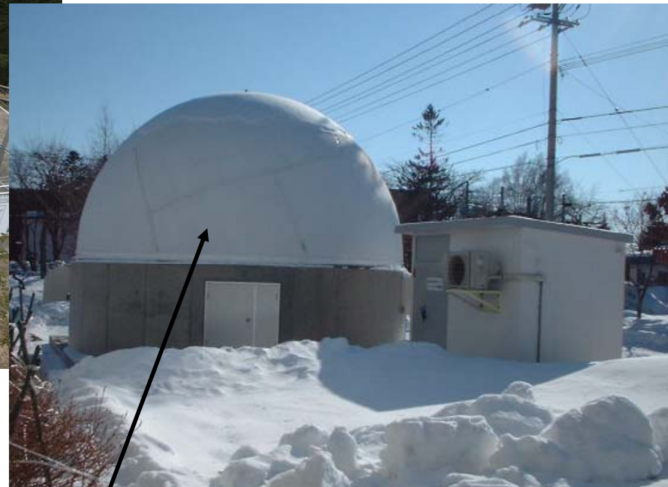
Redome: for antenna protection from snow
